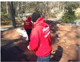
Roof repair on Carolyn Wagner's home
